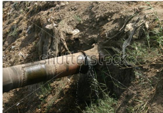
**Figure 2:** Typical water pipe embedded in dirty sand within a dirty environment which will corrodes and contaminates water in the pipe.
