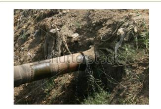
**Figure 2:** Typical water pipe embedded in dirty sand within a dirty environment which will corrodes and contaminates water in the pipe.
